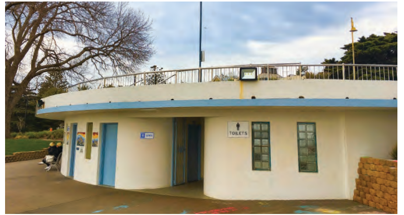
The public toilets on the Cowes Foreshore will be closed until January 2025, when roof waterproofing works are anticipated to finish.
