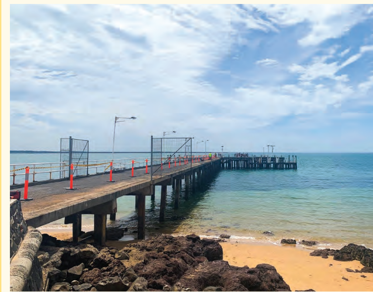
Pile repair work has started on the Cowes Jetty with steel cross beams also being installed. New handrails and asphalt on the walkway are part of the $1.4 million upgrade.
