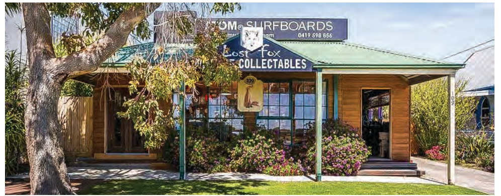
The front dwelling of this 800sqm block is a western red cedar home. Currently the dwelling is being used as an antique shop.
