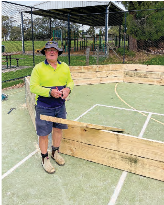
Constructing the new octagonal GAGA pit at Cowes Primary School.
