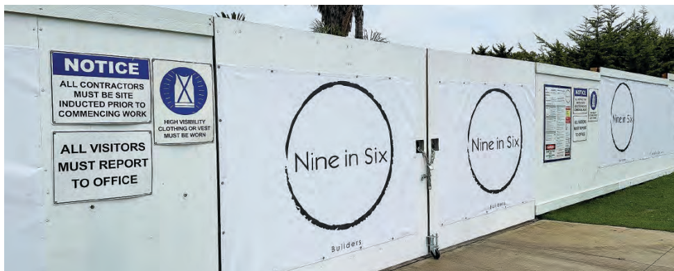
Work on The Block has begun. A shire planning spokeswoman told the Advertiser in 2010 the property was the subject of a development plan overlay, which meant the permit was exempt from public advertising.
