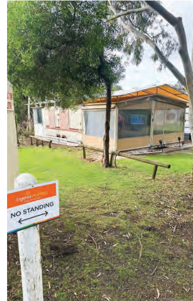
Some annual lease holders at the Ingenia park in Newhaven had to demolish their caravans, after being told they were outside the park boundaries.
